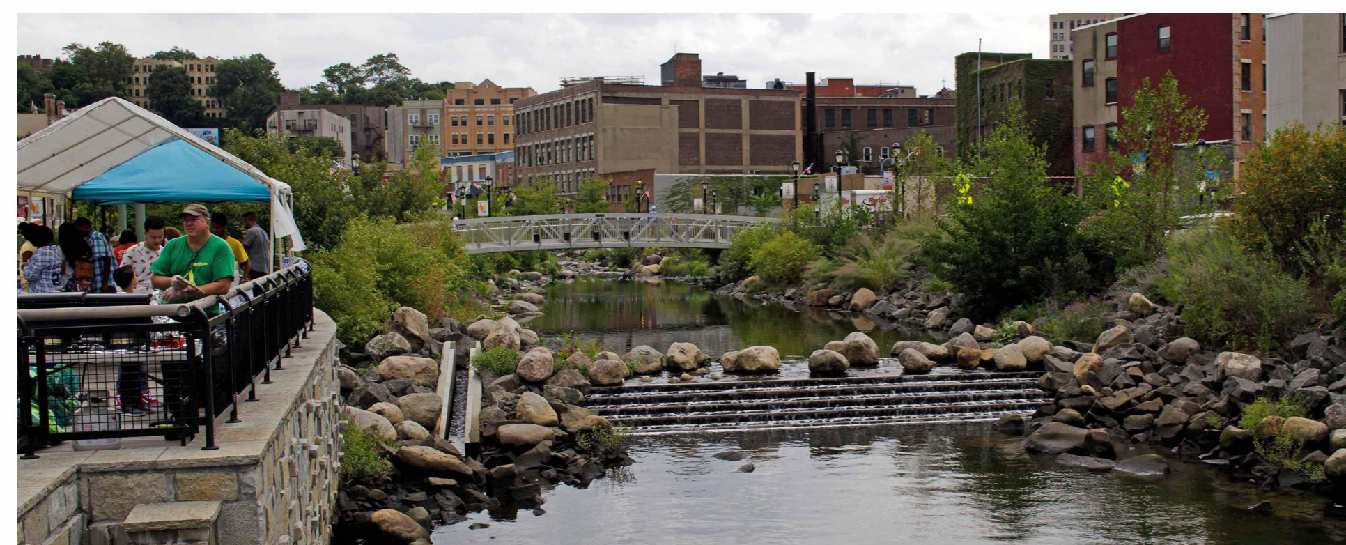
Looking Upstream from the Fish Ladder
