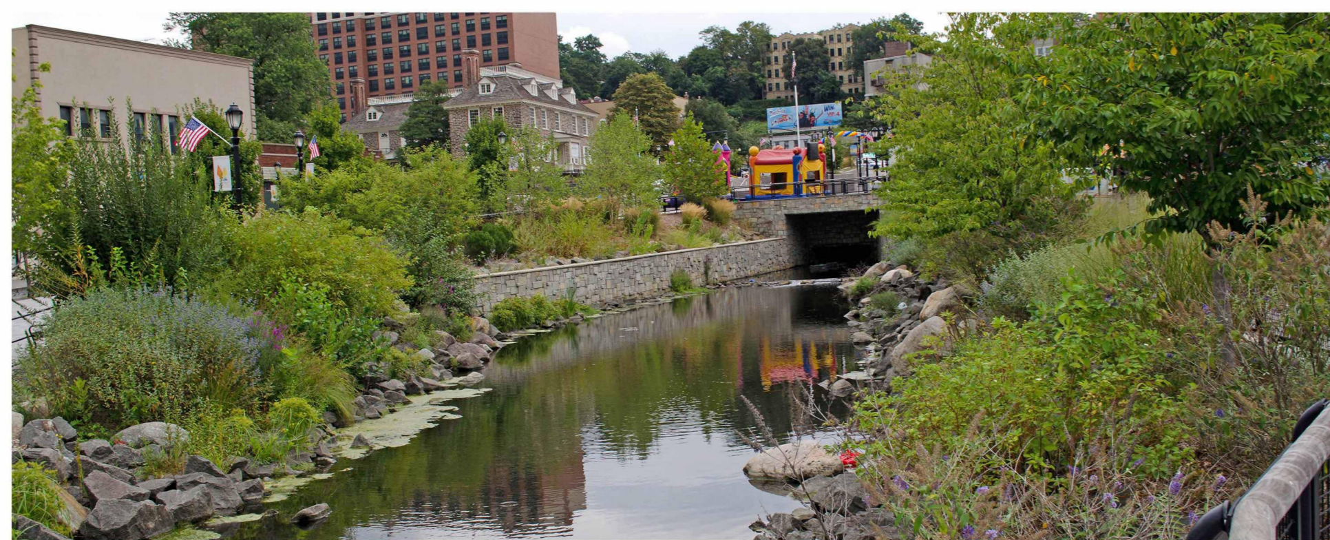
Coming to the Surface
